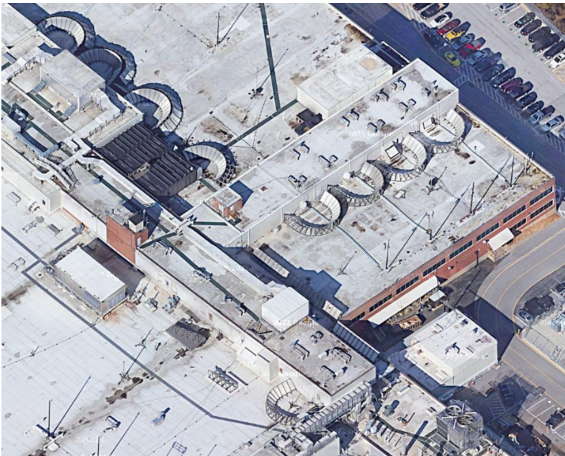
Figure 2. RF Horizons surround the radiating labs on the roof.
