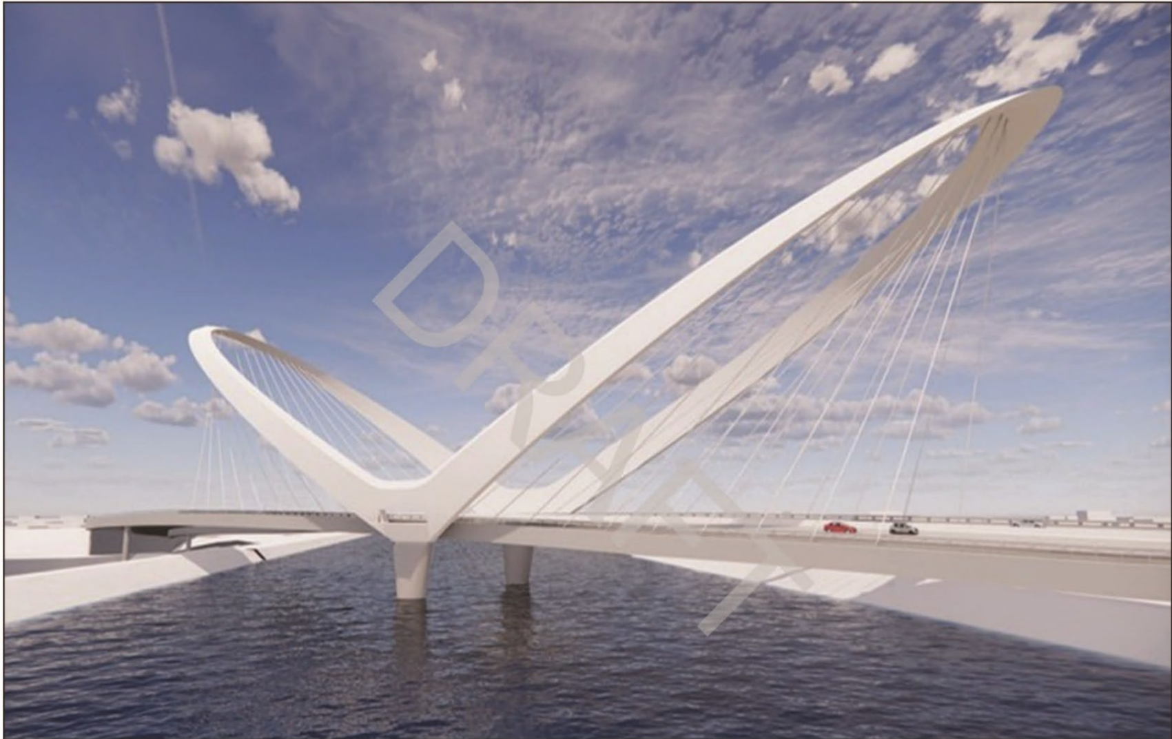
Figure 2: Shoemaker Bridge Symmetrical Rings Cable-Supported Bridge
