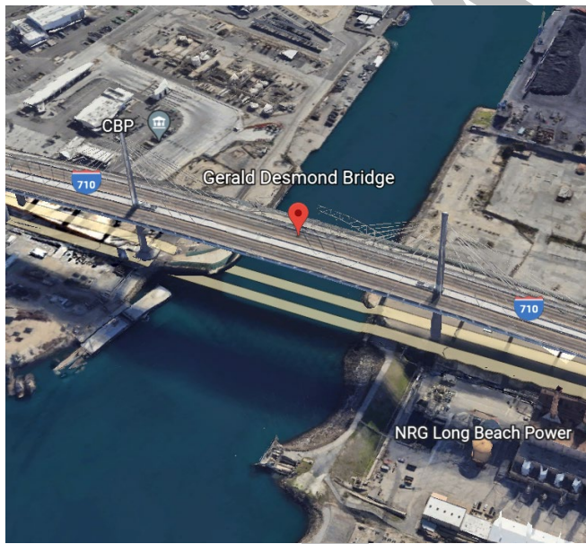
Gerald Desmond Bridge
