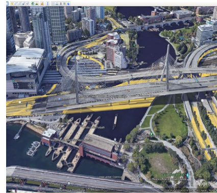
Leonard P. Zakim Bridge Aerial
