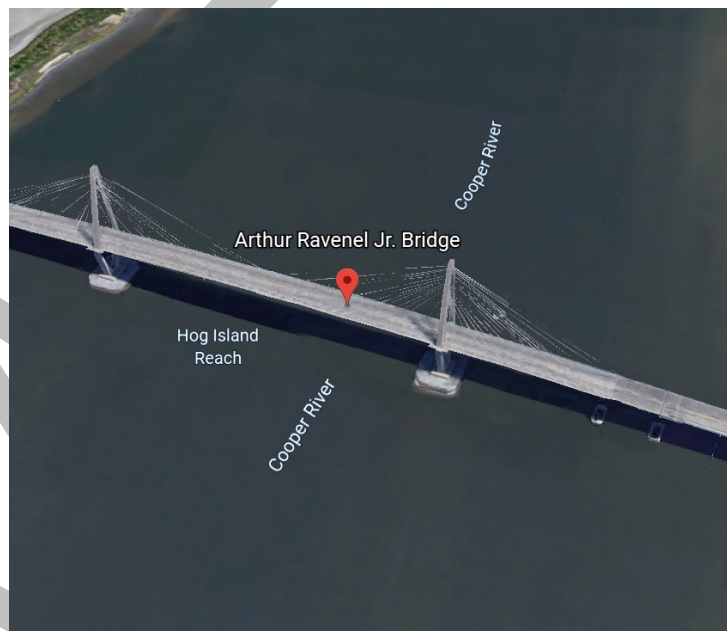
Cooper River Bridge
