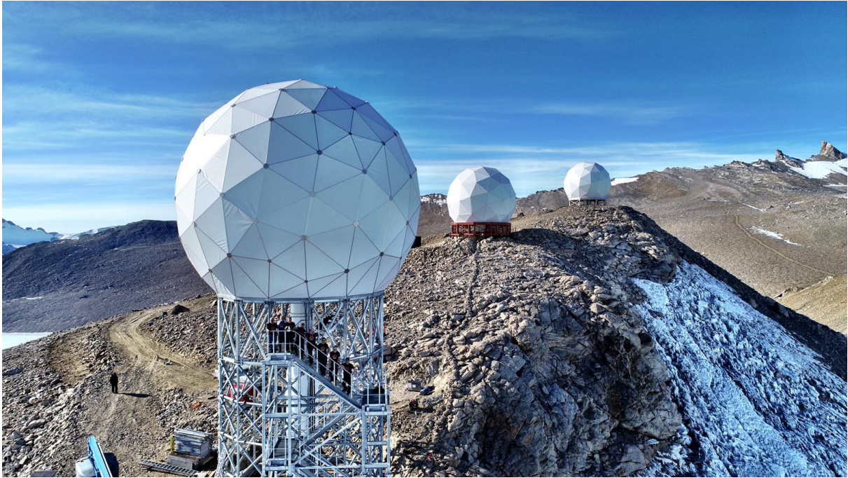
Figure 2 Troll Ground Station with TR9 in front
