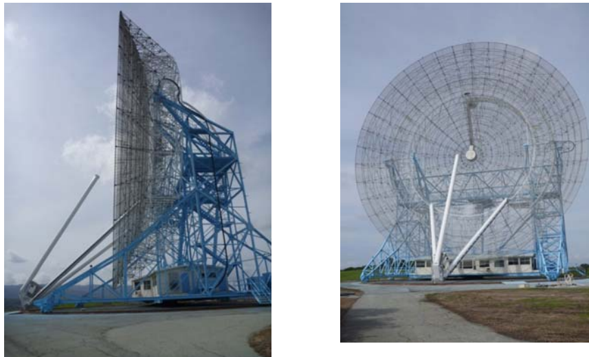
Figure 3. Antenna Tripod in Lowered Position.
