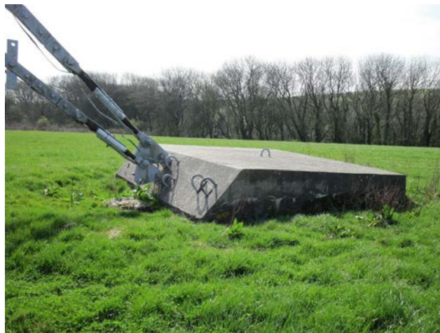
Image 4 Guyed mast guy line anchor
