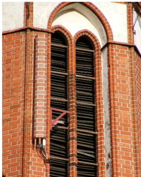
Image 7 A stealth deployment with camouflage
